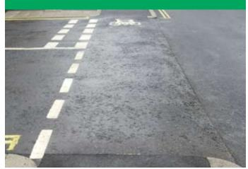
The recent improvements to the Old Shoreham Road in Brighton include a standard detail for providing enhanced cycle priority when tracks run past minor side streets.
